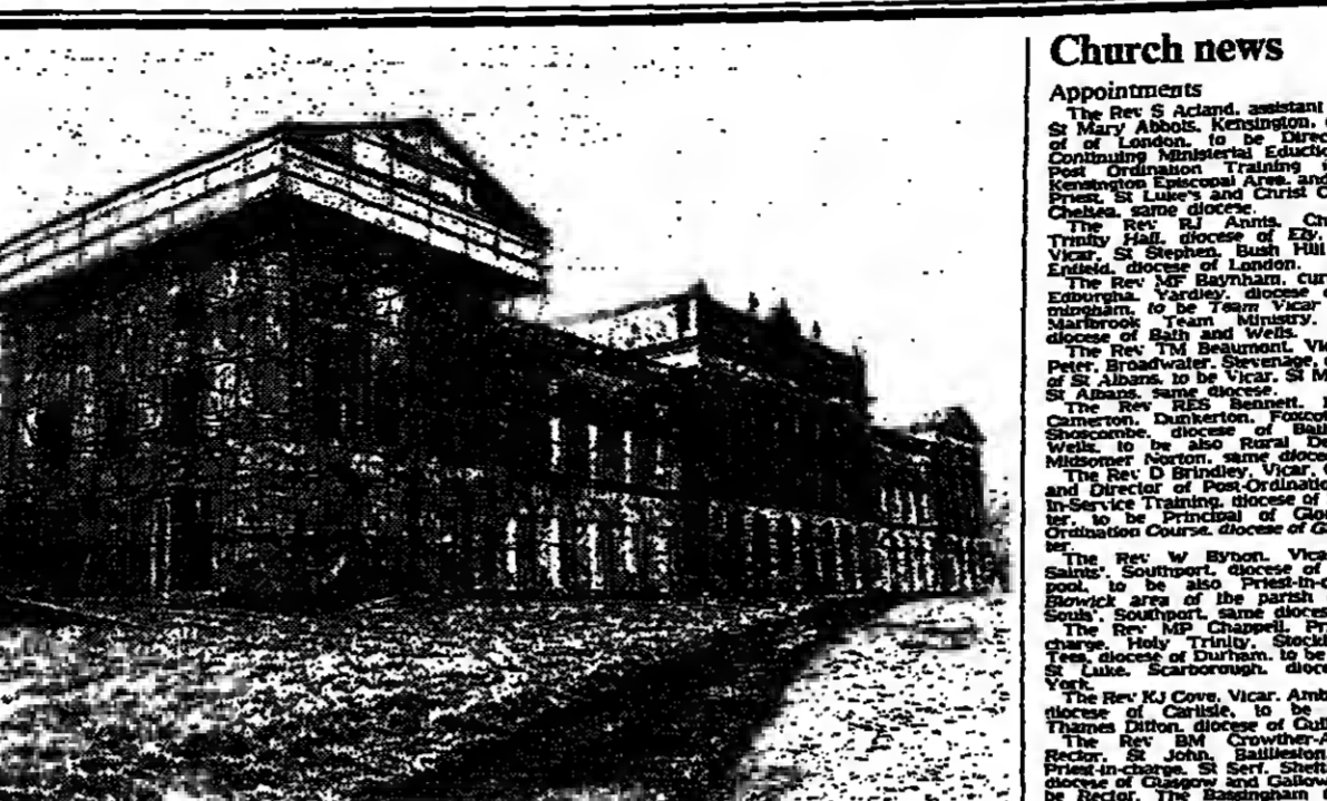
The fine Palladian front of Heveningham Hall in Suffolk under scaffolding (Photograph: Joe McKeown).
